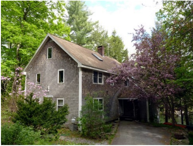
House's North End, facing the road
